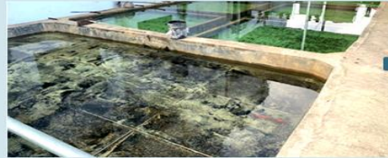
Biological Sedimentation Tank
