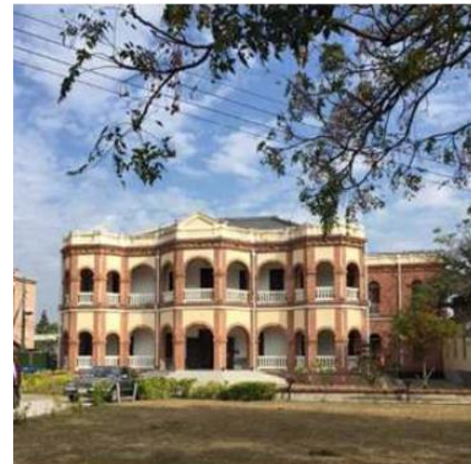
Refurbishment of Taiwan old magistrate's office
