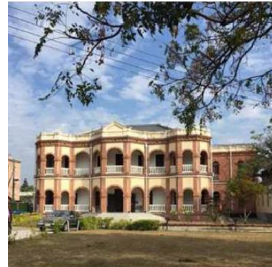
Refurbishment of Taiwan old magistrate's office
